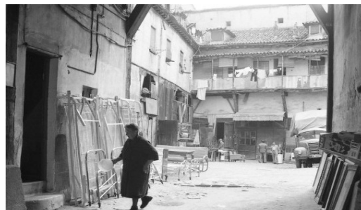
Figure 1. 'Corrala' typical Madrid dwelling: (16th Century) 18 m x 32 m dwellings around a central patio
